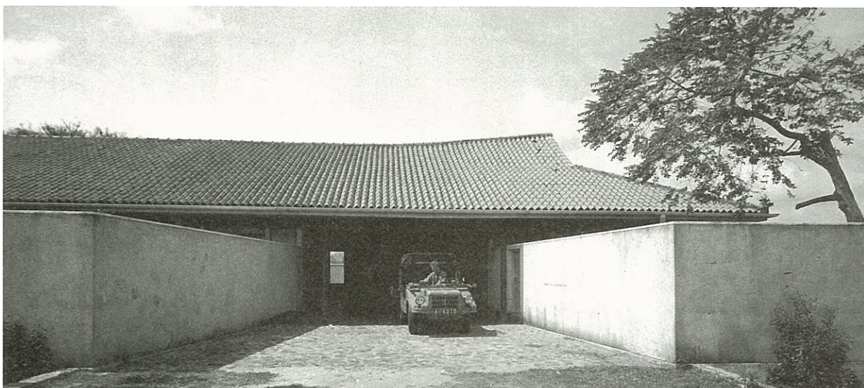
Top: measured drawings of 18 th century trader's house by the coast in Gintota; bottom: the Shell Company District Manager's Bungalow Anuradhapura 1960 – the moment of realisation that the "big roof" is the key.
